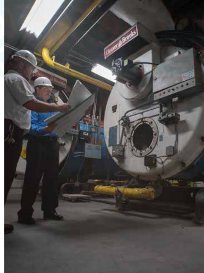
The new boiler stack has to be built before the top floor addition could be shaped around it.
